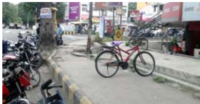
Figure 18 - Rough cuts on walkway in Laxmi Nagar
