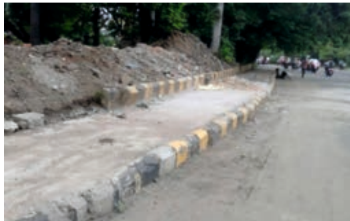
Figure 12 - Walkway under construction at Seminary Hill
